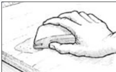
Figure 23 Sand cured fairing compound to desired contour.
