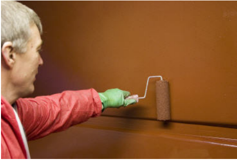
Seaslip is easy to apply with a medium pile roller
