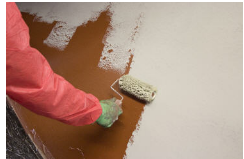
Applying Safeguard TSF with a 7" medium pile roller
