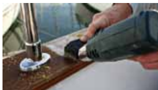
Remove old varnish with hot air gun
