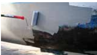
Apply Underwater Primer onto prepared surface
